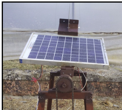
Fig 8. Installation of Solar Tracker Unit on 10 watt photovoltaic panel
